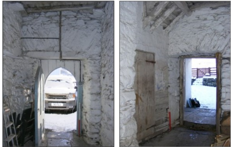
Fig 17. Cross passage: Left - looking towards front; Right- looking towards rear. The door on the left would have led into the hall.-through the 'mell' door. Immediately inside and at right angles to the door would have been a short screen -'the heck'- to protect the fireplace area from draughts
