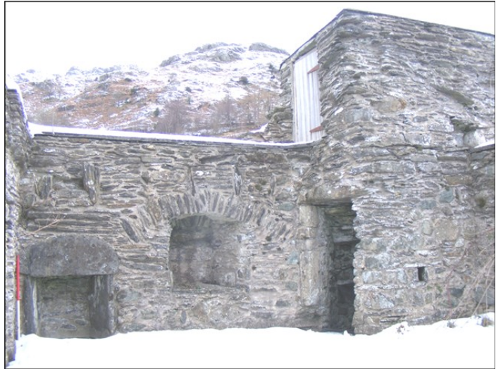
Fig 15: Open 3 rd storey looking North. Note fireplace and window. Garderobe entrance is to left of fireplace. Newel stairs to right with ghost roofline on top (parapet) level.
