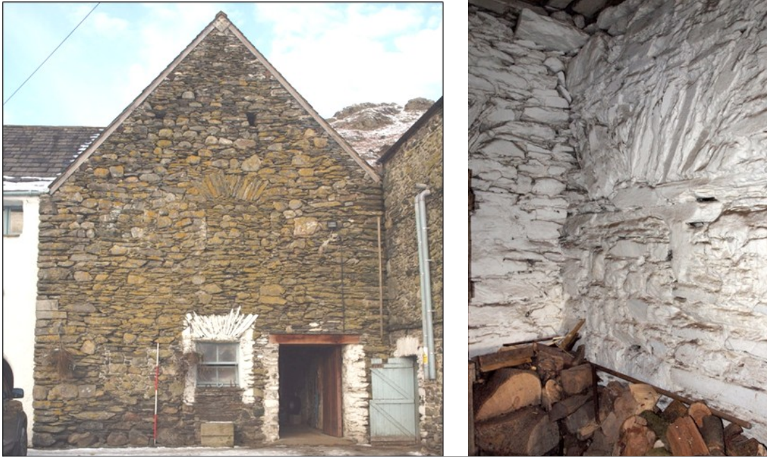
Fig 18: Left: South gable of Chapel Barn cross wing, note large blocked first floor window. Right: Blocked doorway from screens passage into service wing opposite ‘mell door’.
