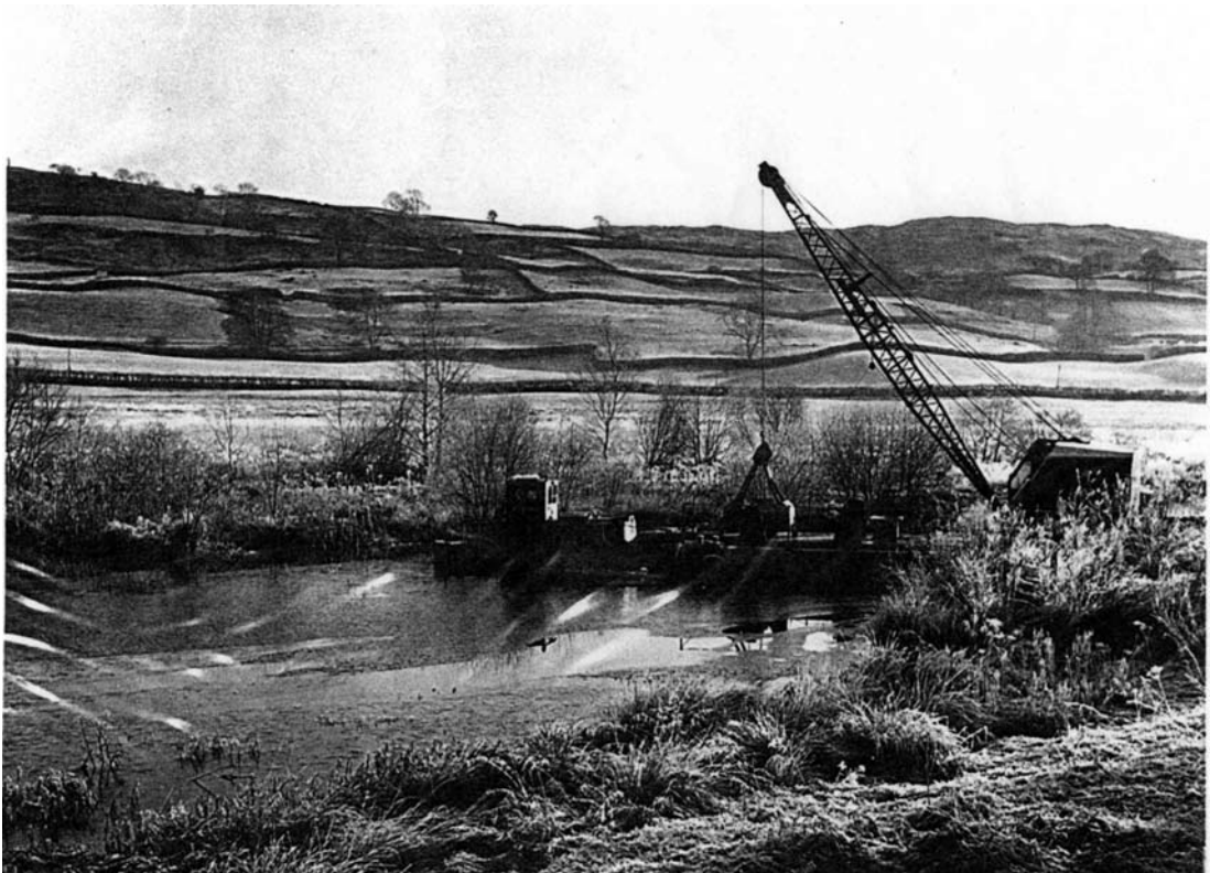
The dredger and barge at work
