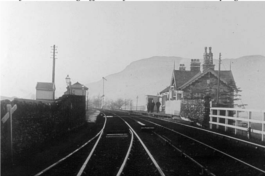
The station crossing where the accident occurred
