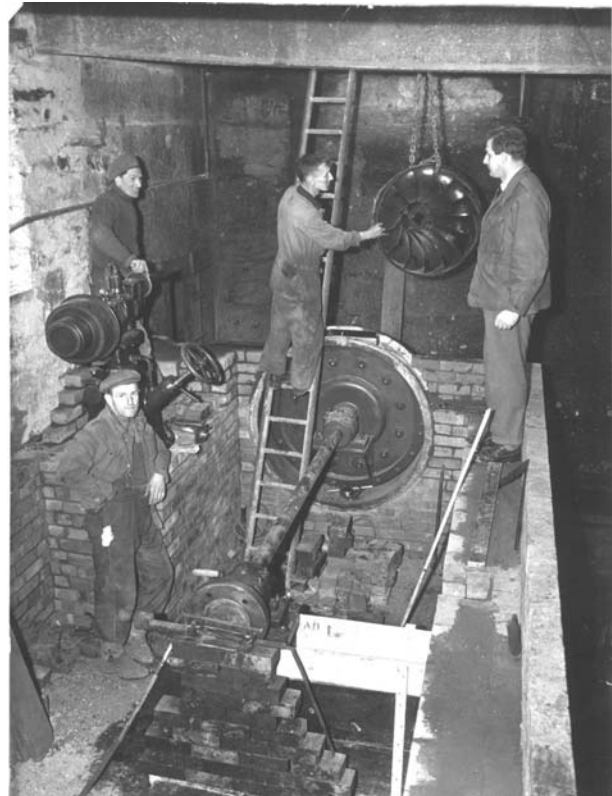
Installing the turbine in 1954
