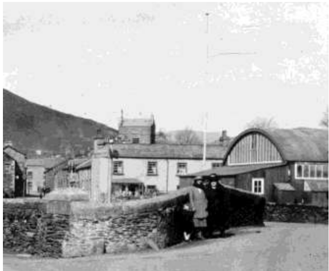
The Drill hall from Gowan Bridge
